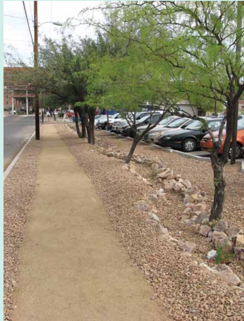
After: A long, thin swale was installed and additional trees and shrubs planted to capture and use runoff from the lot.
