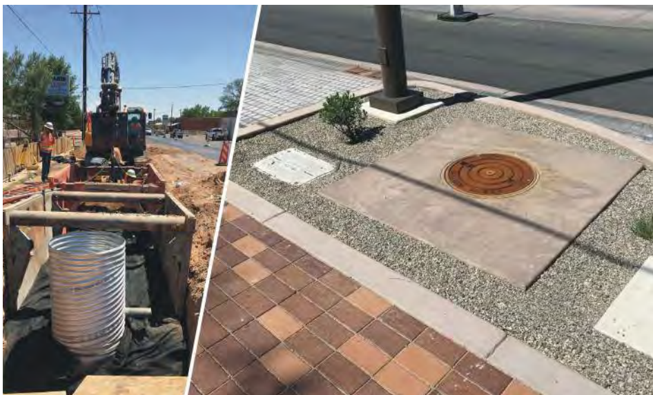
Below grade storage cleanout access during and after construction.
