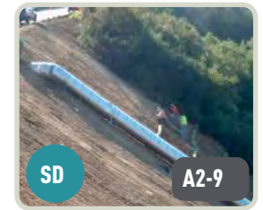
SD A2-9 SLOPE DRAIN
