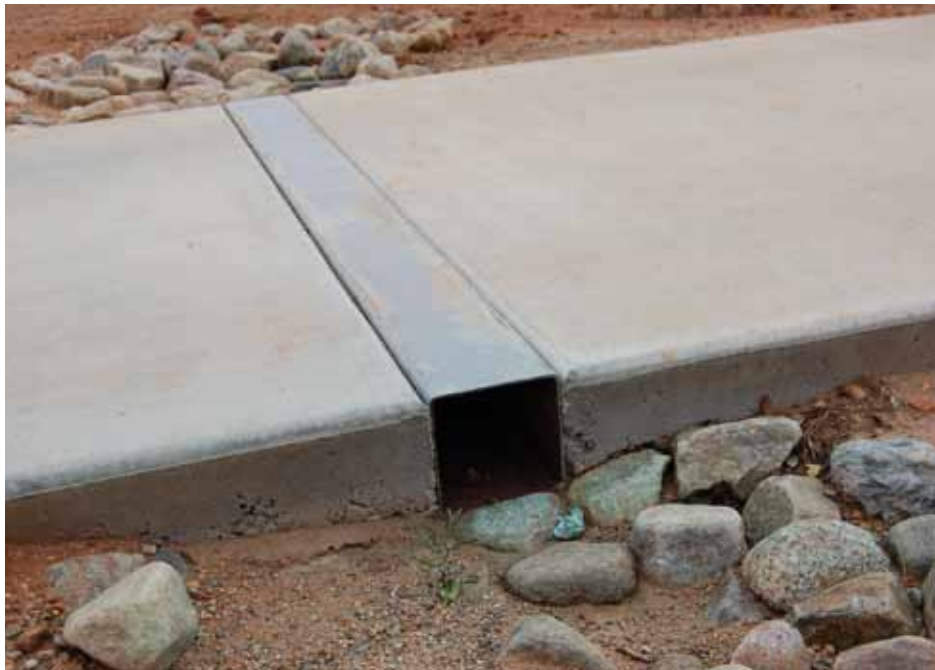
Variations of sidewalk scuppers allowing stormwater to flow under sidewalk.
