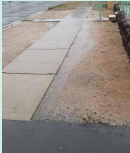
December 2008: Runoff from the lot and adjacent alley wash over bare dirt and the sidewalk into the street.
