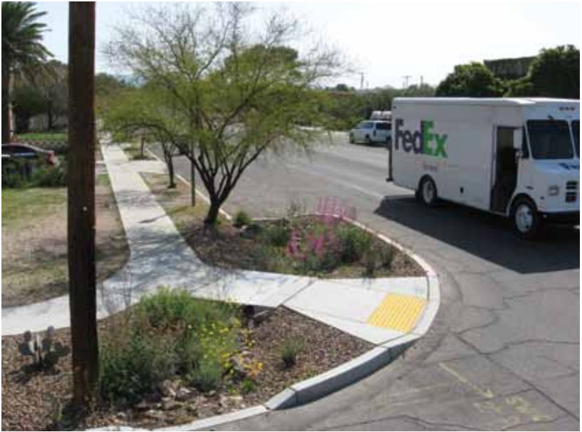
Chicane with no curb cut
