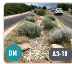
DM A3-18 DEPRESSED MEDIAN
