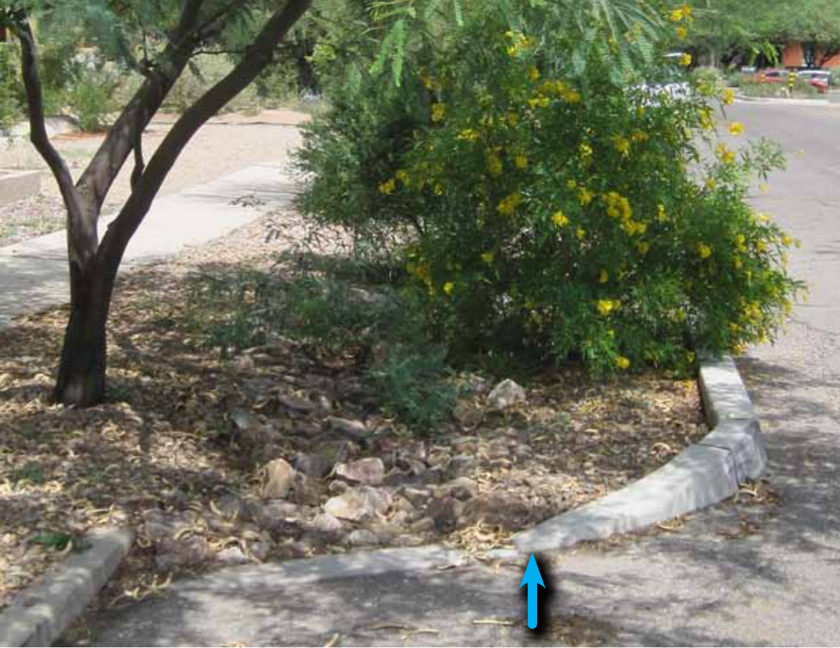
The concrete curb to the left of the blue arrow is flush with the street.
