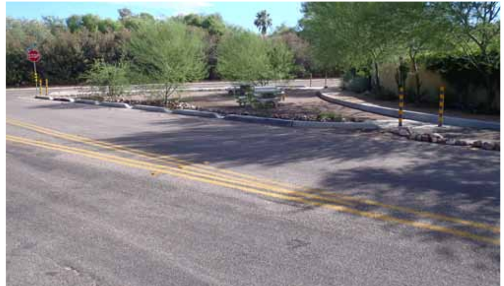
Get creative with your GI. An overwide neighborhood intersection converted into a pocket park is complete with benches and shade trees.
