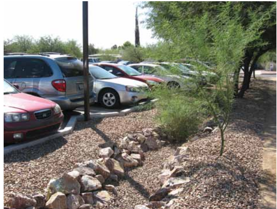
University of Arizona retrofitted their parking lot landscape buffer with a swale to capture runoff.
