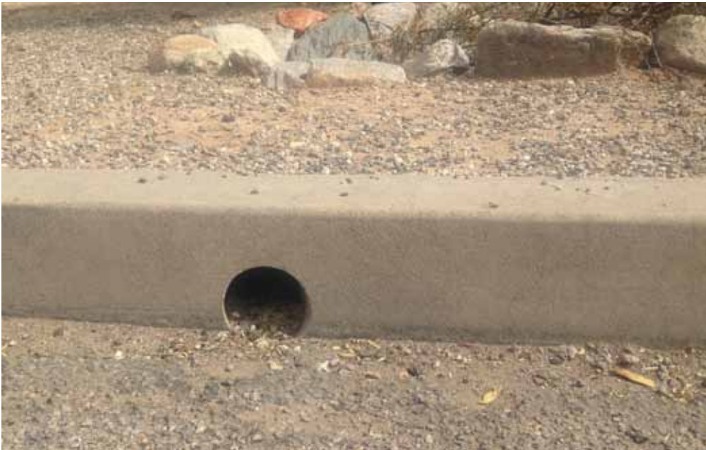
The core inlet is fitted with a plastic pipe sleeve to move water under the pathway into the basin.
