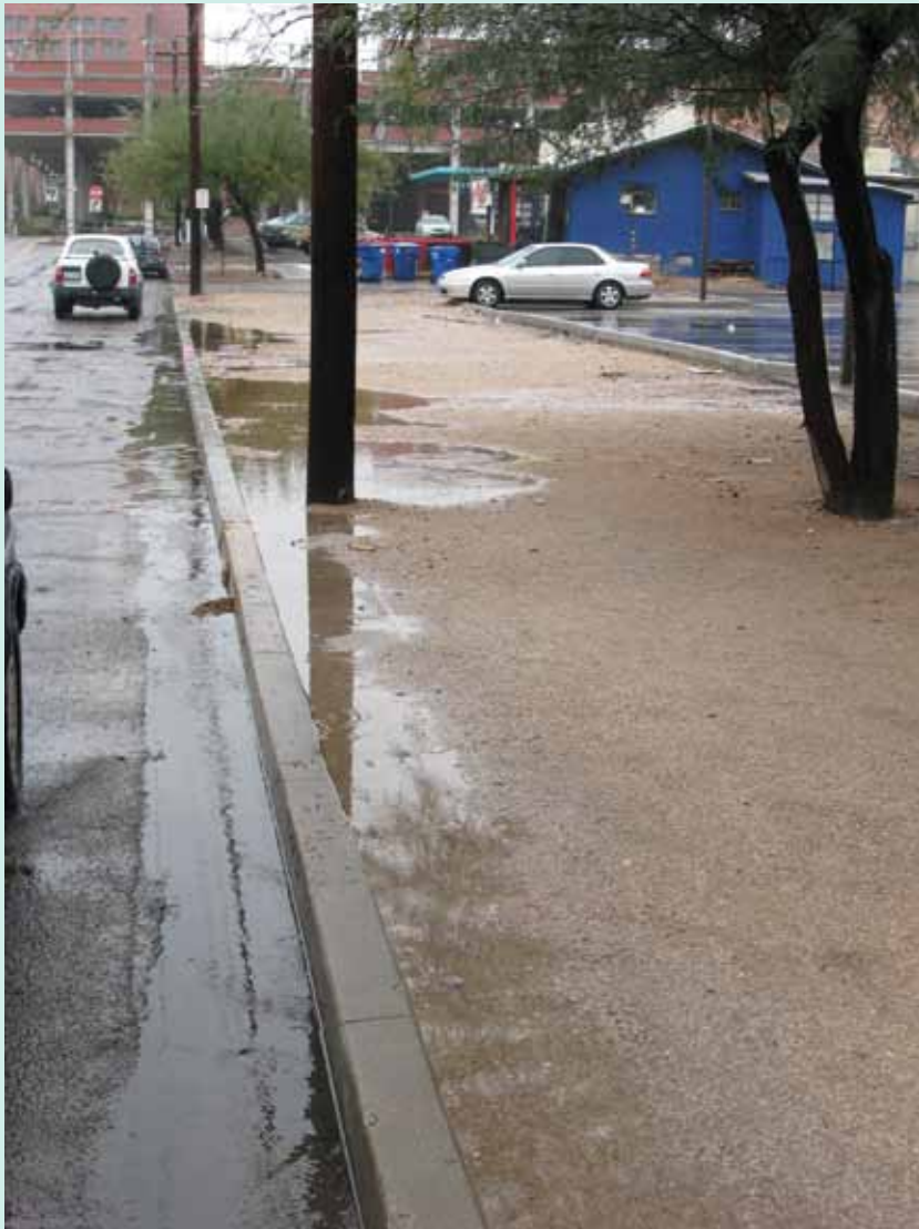
Before: At this University of Arizona (UA) parking lot, small curb cuts allowed stormwater to flow past existing trees onto the pedestrian area in the ROW, and then on to the street.
