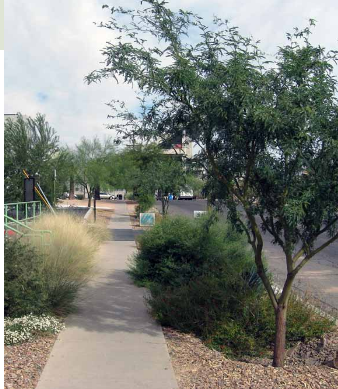
This native mesquite tree thrives in a swale that collects stormwater runoff from the street, providing shade for pedestrians.
