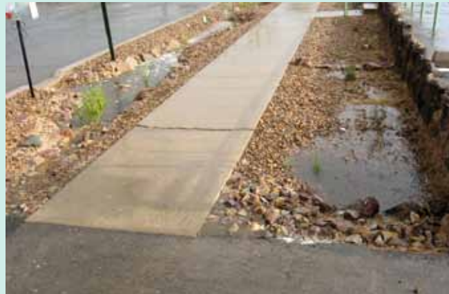
April 2009: newly-dug basins capture storm runoff to feed young plants.
