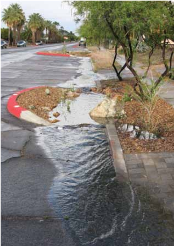
Newly planted chicanes harvest stormwater moving along the gutter. Right: This stormwater basin is constructed with repurposed urbanite in La Paz, Mexico.
