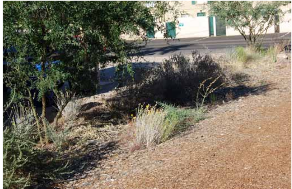
A small basin accepts and infiltrates more street stormwater runoff than is needed to irrigate these native plants as highlighted in the adjacent table.
