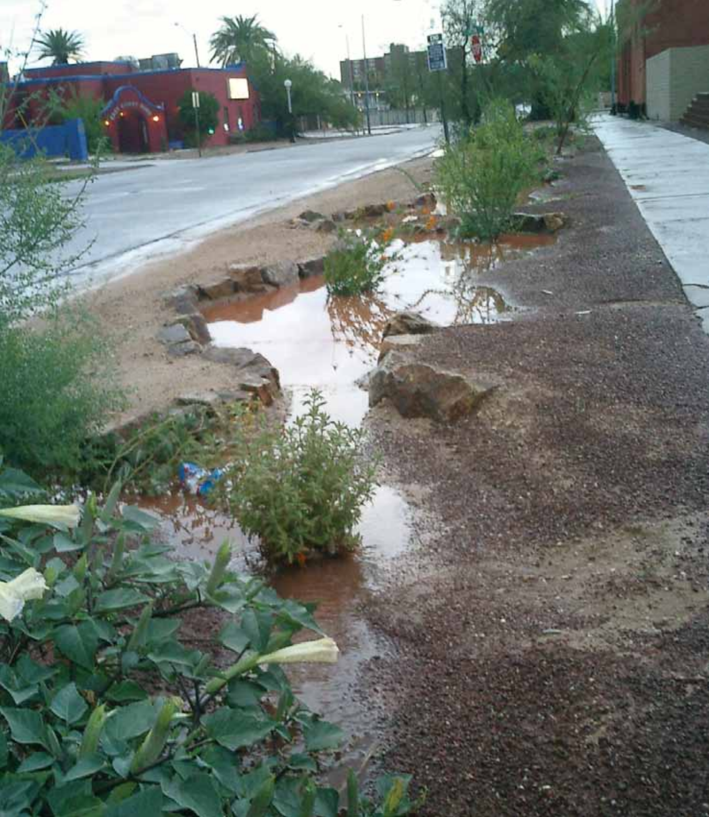
This series of basins collects stormwater from the adjacent sidewalk and businesses (without curb cut).
