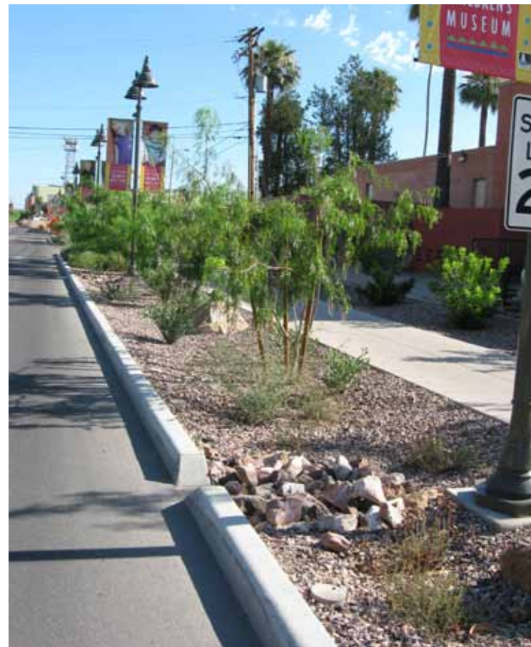
This long, shallow swale in the right of way has multiple curb cuts along its length.
