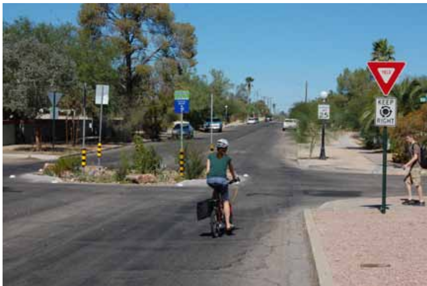
A green infrastructure traffic circle thrives with native plants, directs cyclists with signage, and calms neighborhood traffic on overwide streets.
