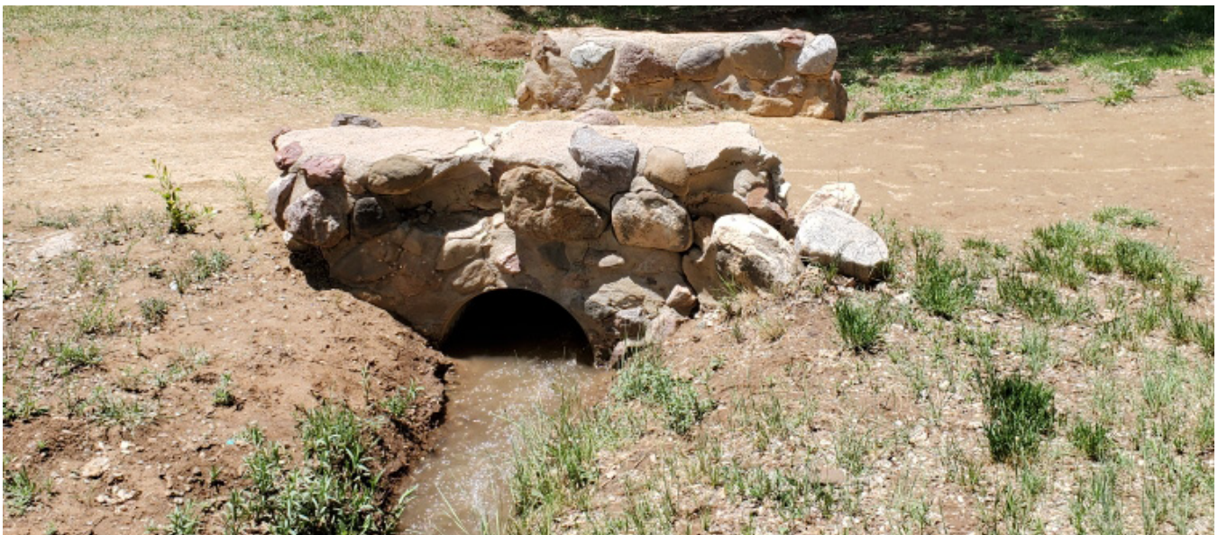
Acequia flowing through Kit Carson Park. Courtesy of GWS.
